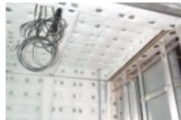
FyreWrap Marine Blanket is made with Insulfrax fiber and is USCG Approved
